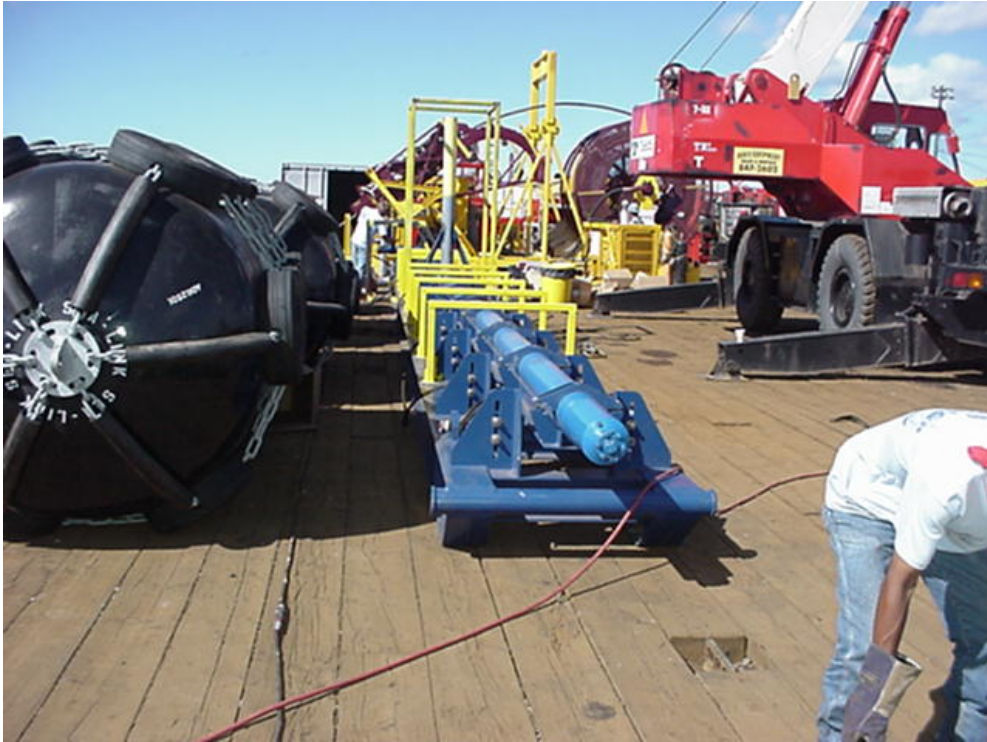
EQUIPMENT TRANSPORTED ON CMS 250 BARGE
