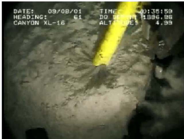
Figure 5-40. Suction Hose Removing Bow Sediment.
